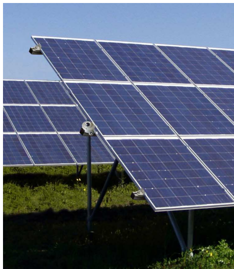
Example of positioning of the pyranometer
